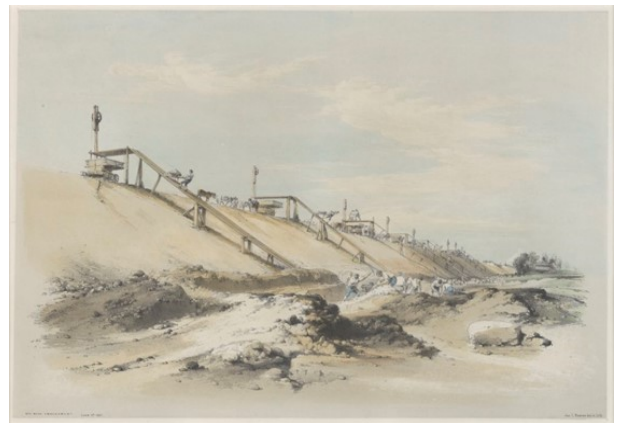
The method of making the shallower type of cutting
